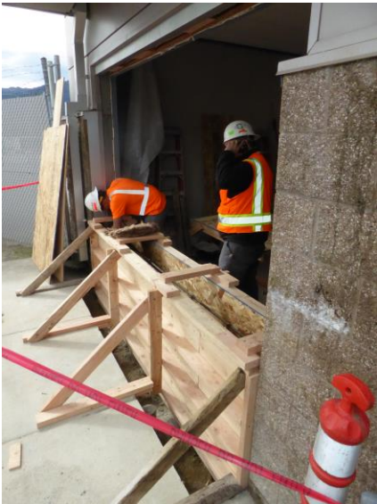
Terminal East Wall Infill
