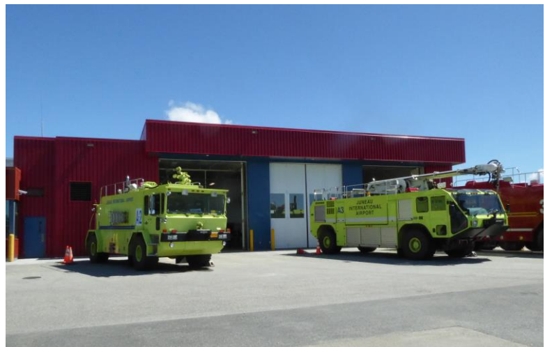
West elevation of ARFF apparatus bays.
