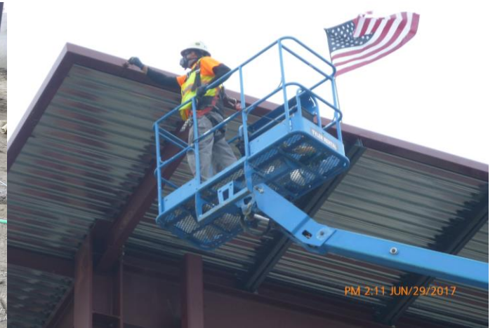
SREB: F&W carpenter applies primer to steel at roof eave.
