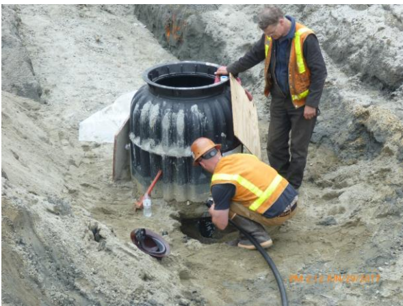
Coogan Construction workers connect sewer line to lift station.
