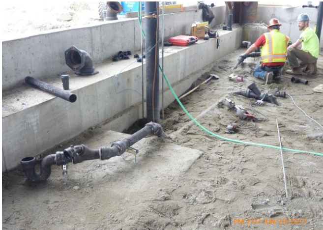
SREB: Harri Plumbing & Heating workers install underground plumbing lines.
