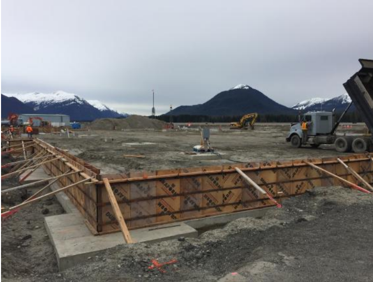
View of SREB construction looking toward Southeast.
