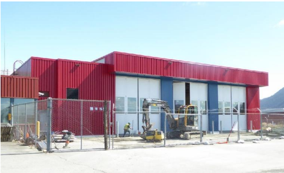
West elevation of ARFF Apparatus Bays.
