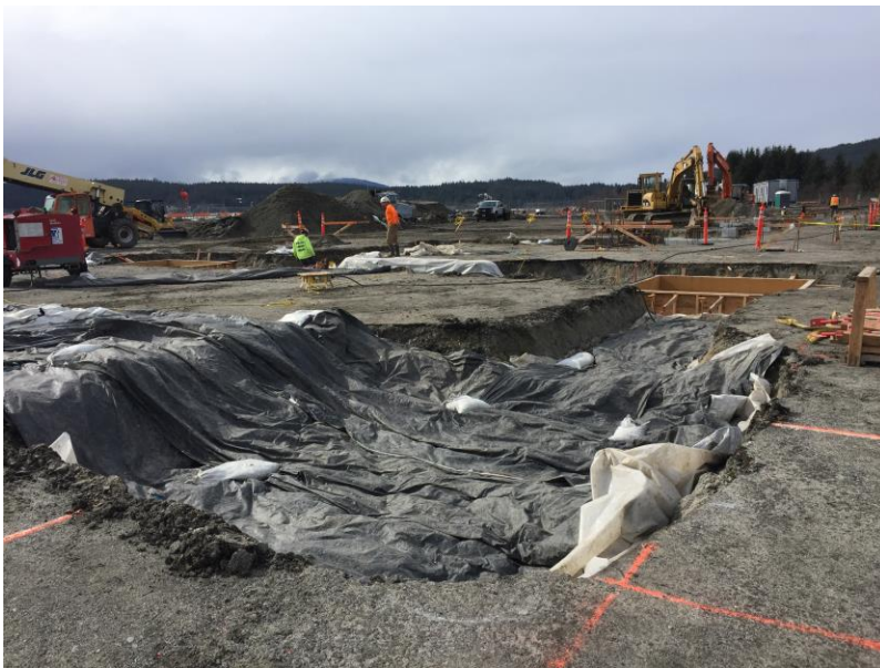
SREB foundation work continues.
