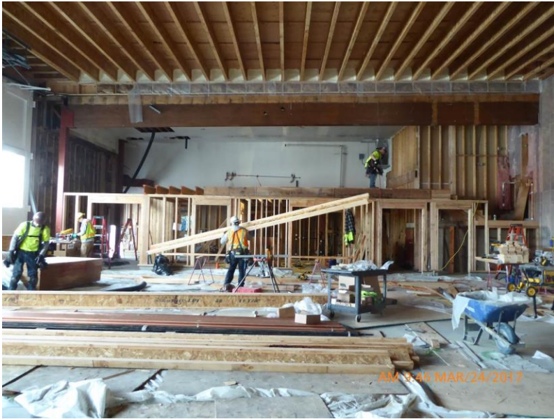
ARFF Station floor mezzanine framing underway.
