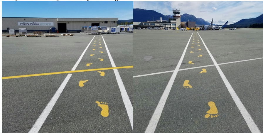
Sample main ramp walkway marking
