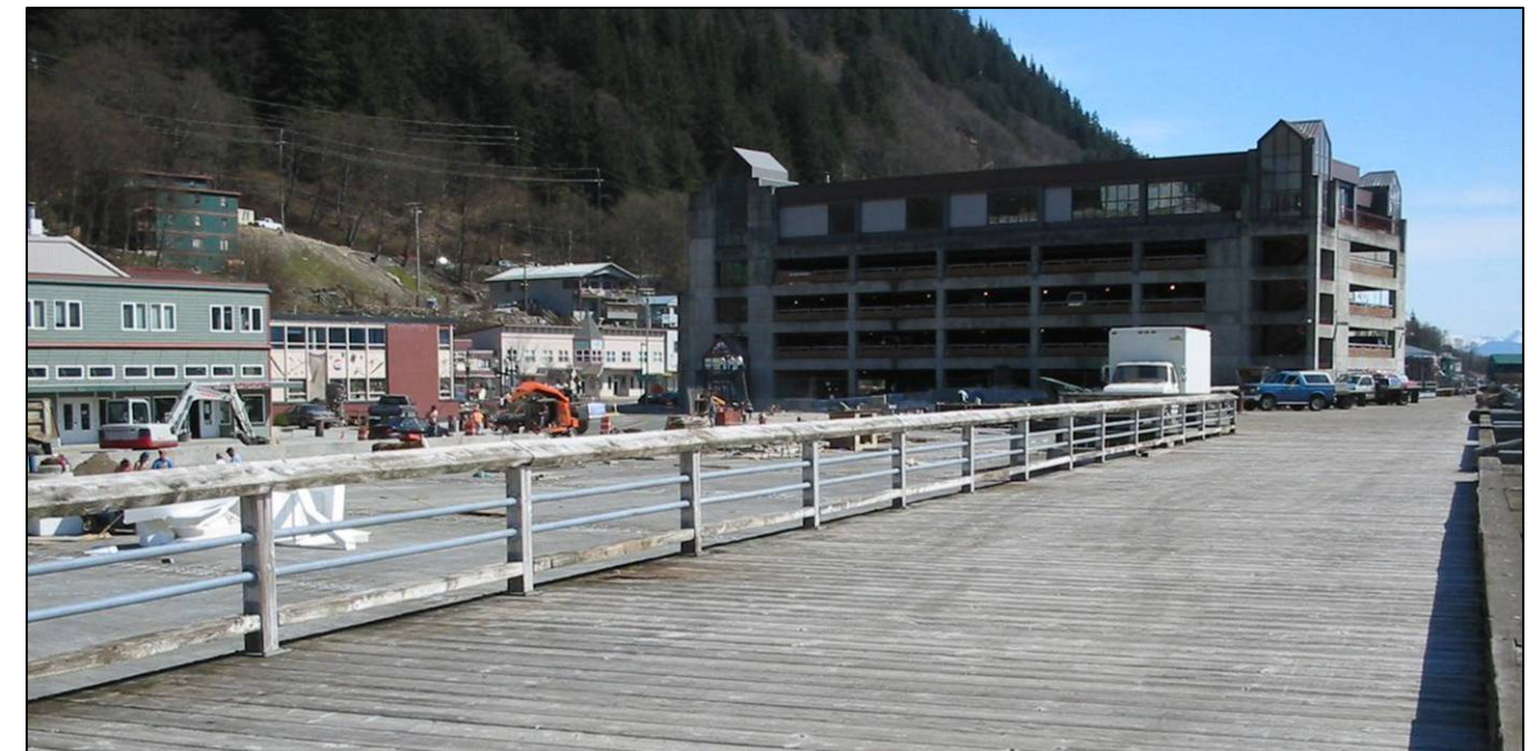
View of the Steamship Wharf and the Juneau Public Library/Parking Garage (Area C)
